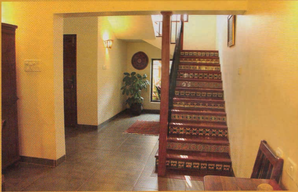
the timber staircase with handmade tiles from Mexico used as risers and a Spanish style handrail
