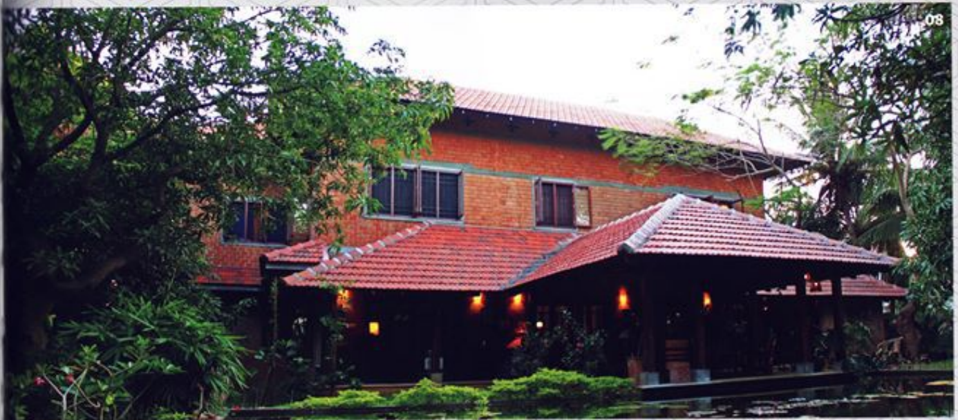
09 | The roof is a predominant feature in the elevation.
