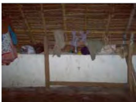
Low Brick Wall
