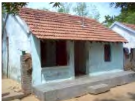
Mangalore Tiled Roof
