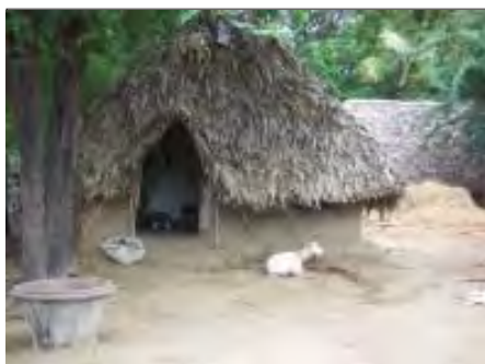
Low Mud Wall and Palm Thatch Roof
