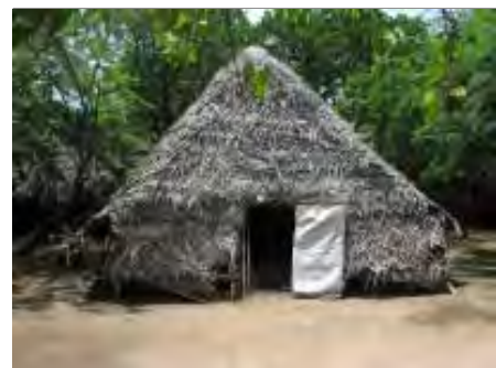
Coconut Thatch as Walling and Roofing Material
