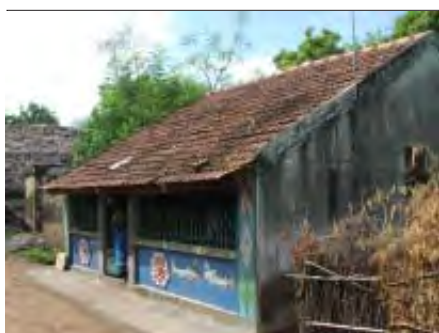
Verandah Enclosed into a Room
